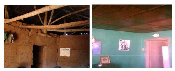
**Figure 5.** A) Habitat showing a lot of space between the rough wall and the roof with several cracks in the wall (Dangbo); B) habitat with a ceiling and smooth wall without cracks or spaces (Dangbo).
