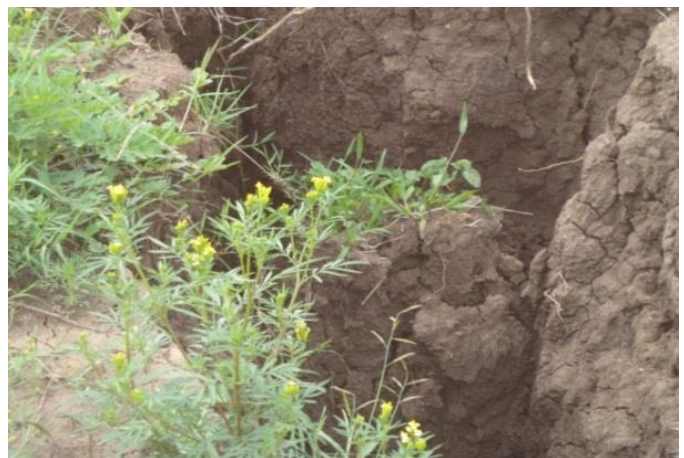
Figure 7. Unstable outer bank showing cracks. Monene, 2014: Photographs were taken 10 m downstream of Kangundo Road Bridge on 17/12/2013.
