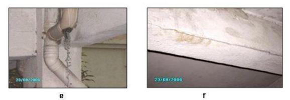
Figure 3. Façade and services defects at post occupational stage.
