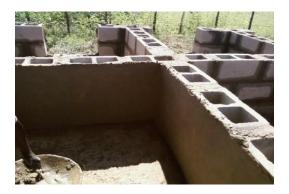
Plate 18. Compost cells under construction.
