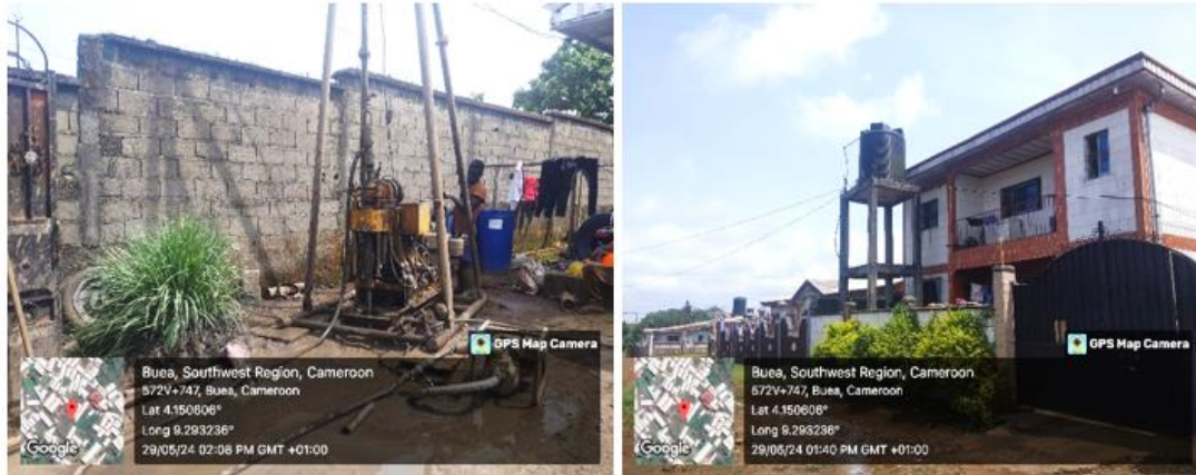
Figure 6. Sample boreholes in Buea. A) Borehole construction; B) Already constructed Borehole (MissBright Bomaka) with a tank (Kawah-Bomaka))
